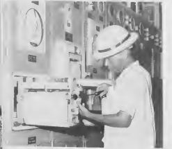
ELECTRONIC TEMPERATURE retractor at the Cat Cracker gets field repairs from E. Geerman, instrument mechanic A. REGISTRADOR electronico di temperatura na Cat Cracker ta worde drecchi den teld door di L. Geerman, instrument mechanic A.
